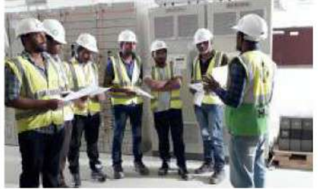
66/11kV Khalifat -2 Substation
