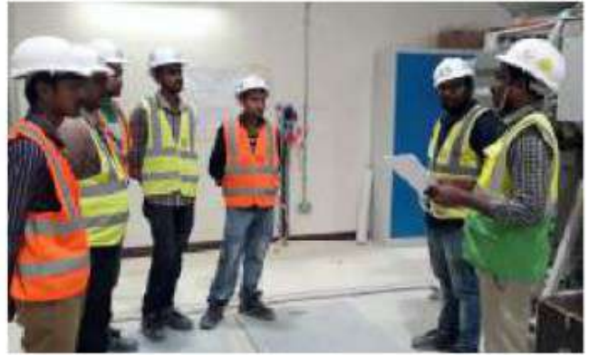
132/11kV Umm Al Hou-2 Substation
