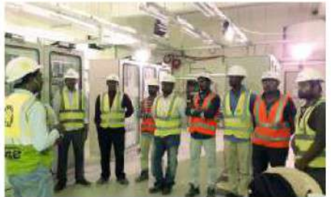
66/11kV Murrah South Substation
