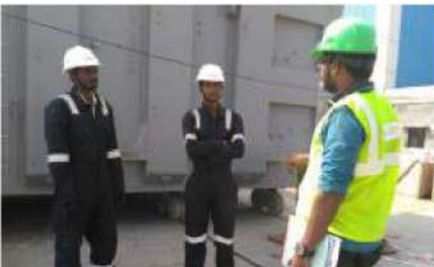
HVDC Pugalur (Transformer area Pole 1)
